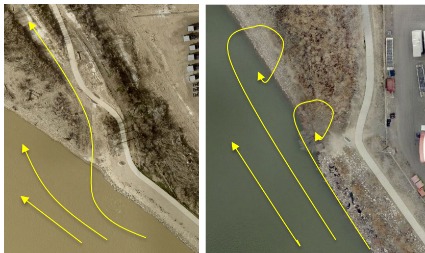
Figure 6-8. (Left) Bank armoring that transitions to a side channel where flood energy is naturally dissipated. (Right) Abrupt end of bank armoring with bank erosion occurring downstream along unarmored bank. Yellow lines indicate hypothetical flow paths.
