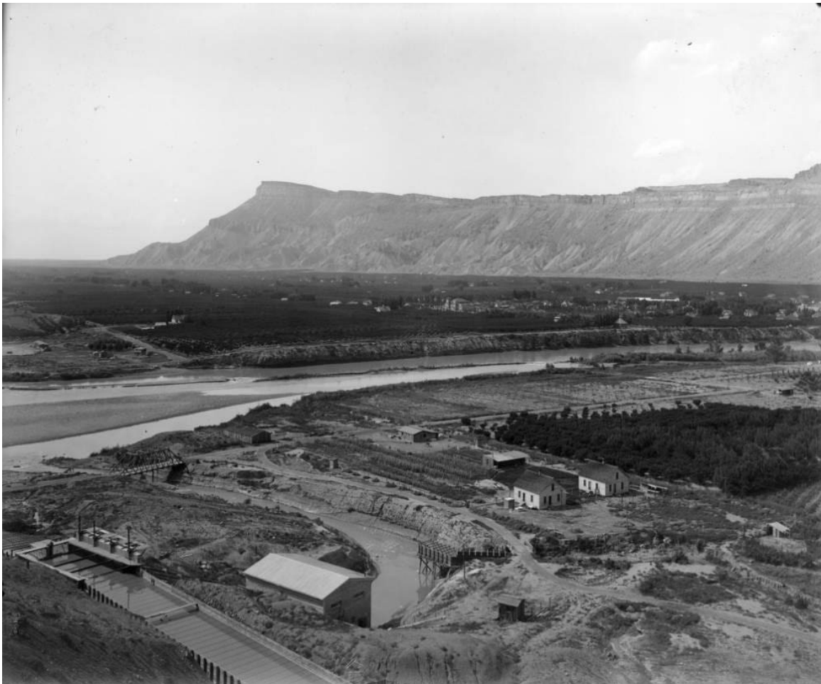
Figure 4-3: Early 20 th century (~1912) image of diversion system along the Colorado River near Palisade, CO (Denver Public Library).
